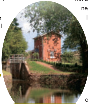
Oxenhall Lock and Lock Keeper's Cottage
